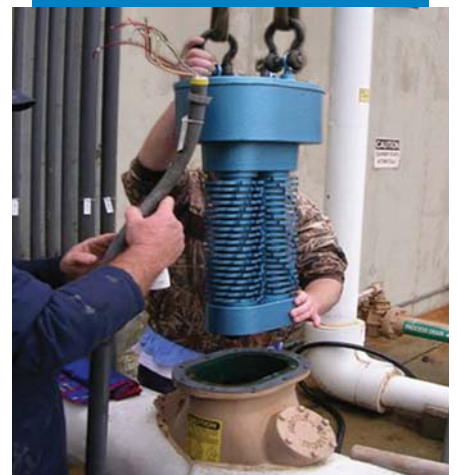
Moyno Edge replacement grinder cartridges are designed to fit within the Muffin Monster® grinder housing, providing a higher level of performance at an economical cost*.
